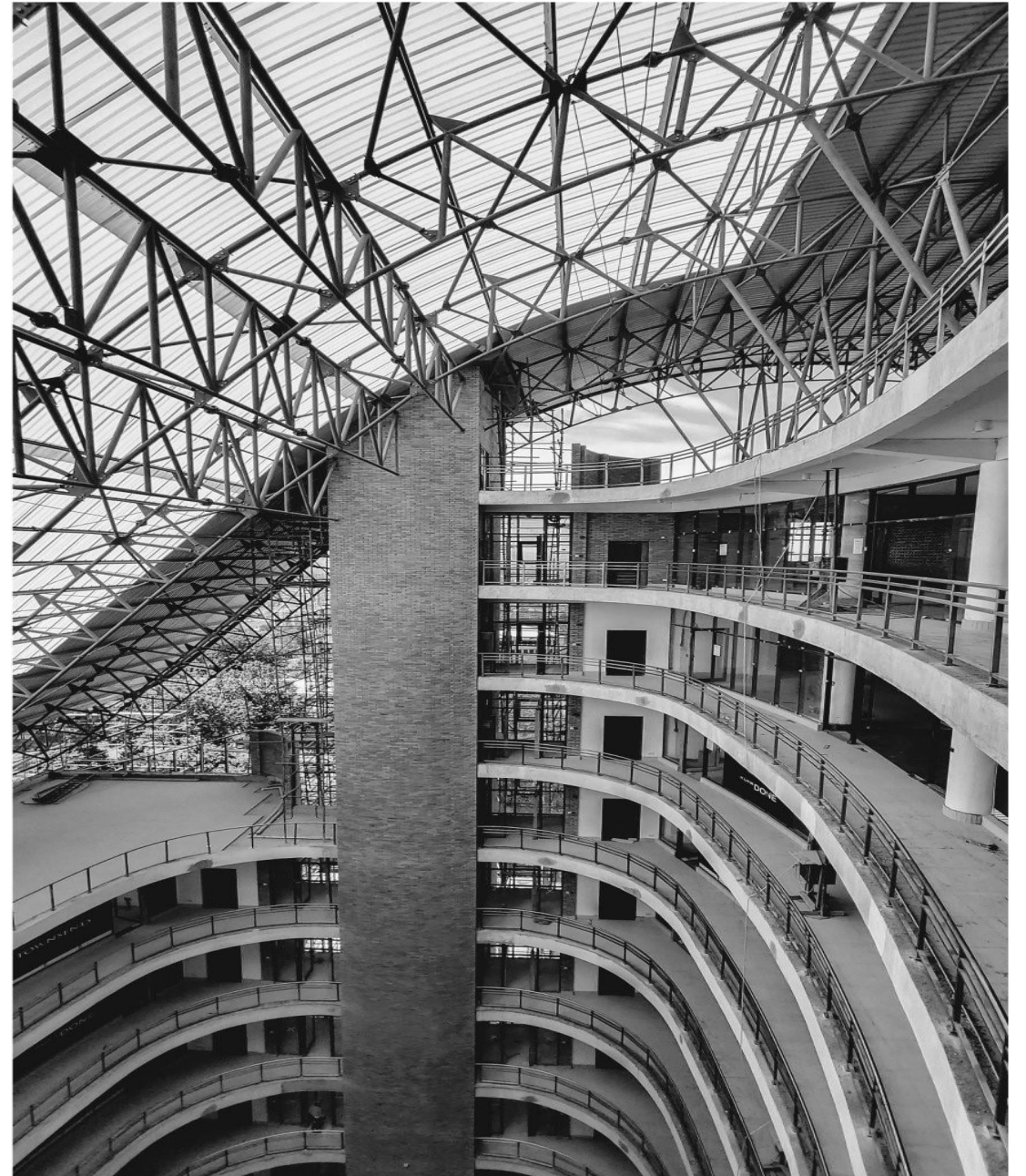
I & M Building
